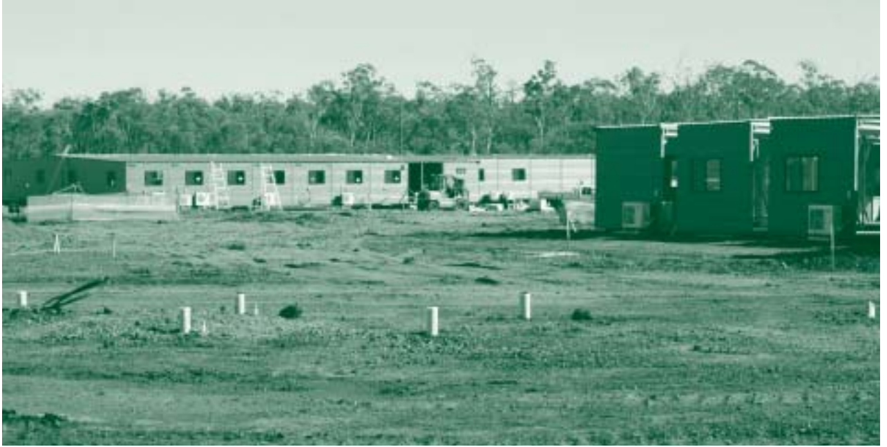
The accommodation village has been under construction at Clermont Mine.
